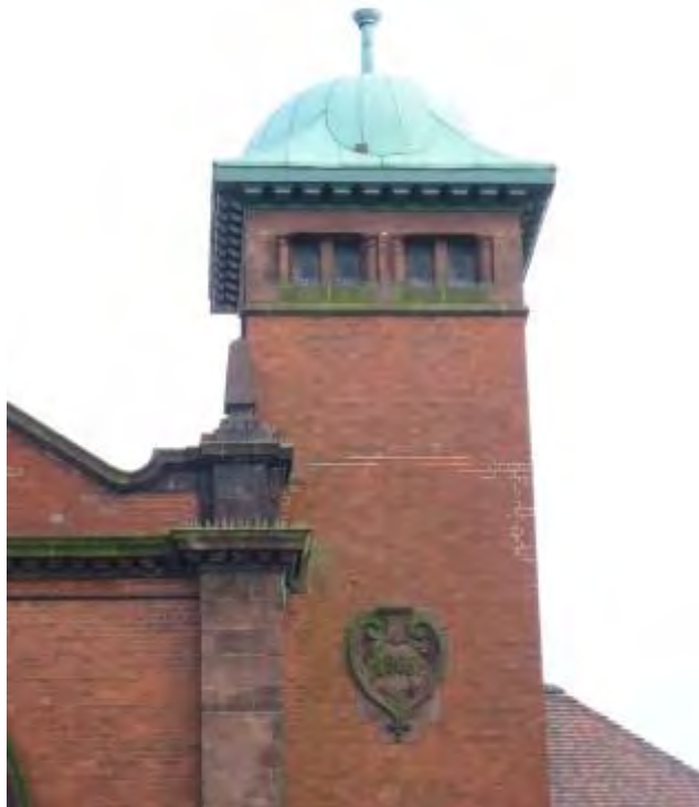
Fig.17: Copper dome roof on Burslem United Reformed Church, Moorland Road
