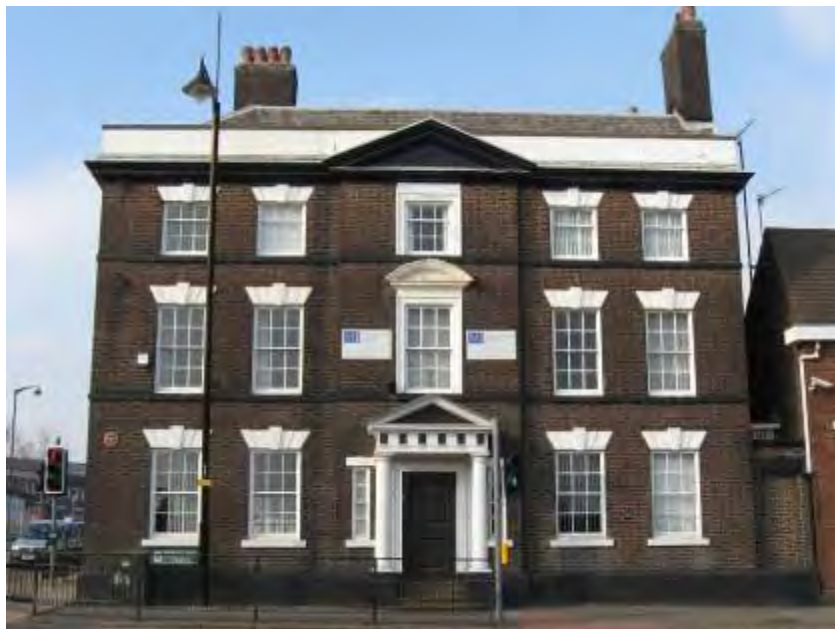
Fig 21: Moorland House, Moorland Road (Grade II* listed building)
