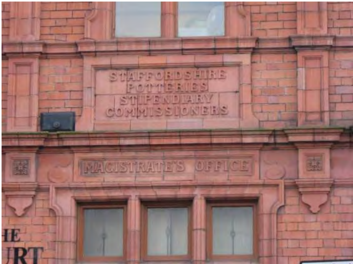
Fig 13: Terracotta Detail, Moorland Road
