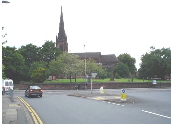
FIGURE 3: Holy Trinity Church and the junction of Hartshill with Princes Road. Landmark, node and focal point.
