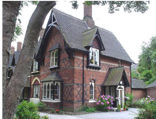
FIGURE 9: Patterned brickwork. (Above) 10 Wilfred Place; (top right) Flemish bond 38-42 Queen's Road; diaperwork (left) at Minton Cottages.
