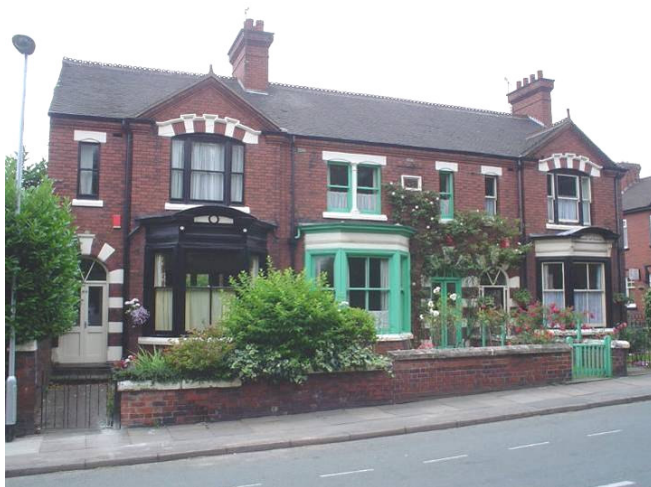
FIGURE 13: A surviving range of historic windows 30-34 Queen's Road. Note low garden wall, front gardens and use of moulded brick.
