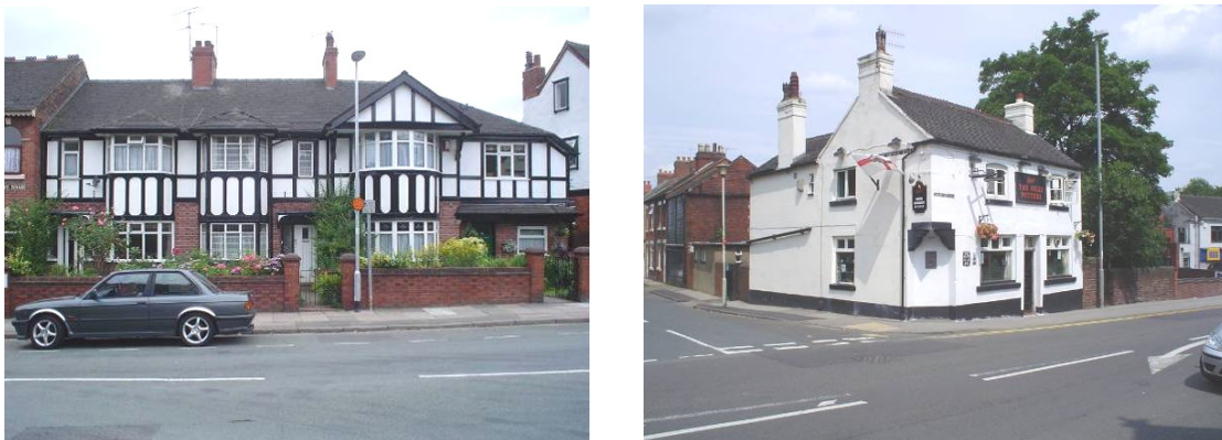
FIGURE 11: Façade finishes. (left) Flemish bond brick with render and half-timber cladding 2-8 Queen's Road; (right) flat render at the Jolly Potters.
