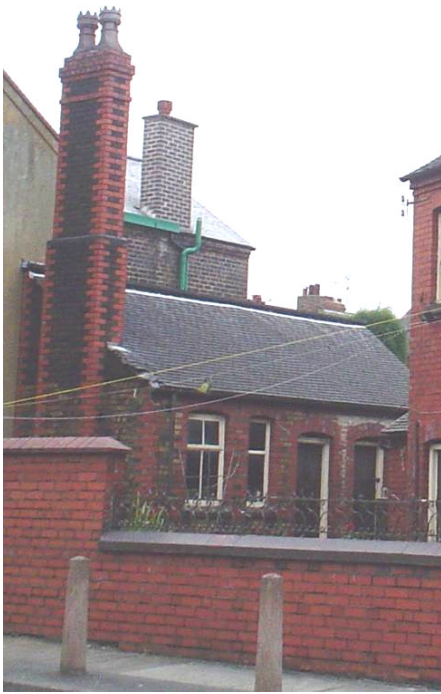
FIGURE 9: Patterned brickwork. (Above) 10 Wilfred Place; (top right) Flemish bond 38-42 Queen's Road; diaperwork (left) at Minton Cottages.
