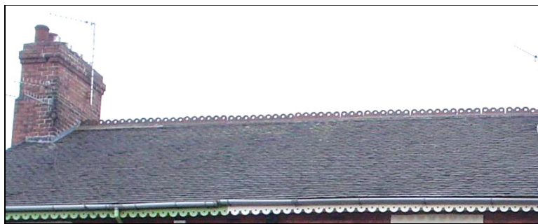
FIGURE 12: Ridge tiles and bargeboards in Queen's Road. Tiles are the Area's typical roofing material.
