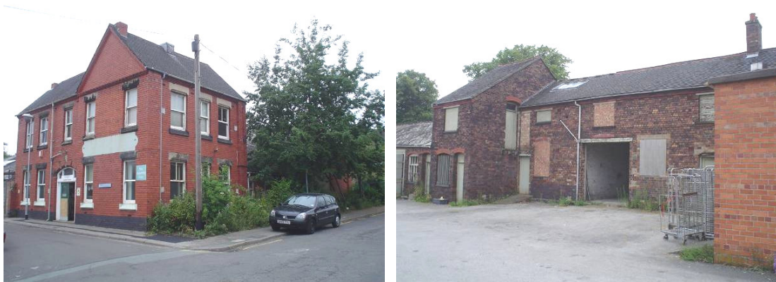
FIGURE 20: Buildings of the former North Staffs Territorial Association. (left) Office with painted sign – the drill hall is hidden by trees to its right. (right) Stable blocks behind drill hall.
