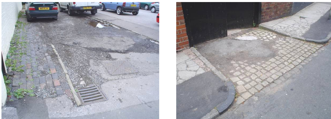
FIGURE 17: Historic street surfaces. (left) Hulme Street; (right) an access on Vicarage Road with curved granite corner pieces to the kerbs.
