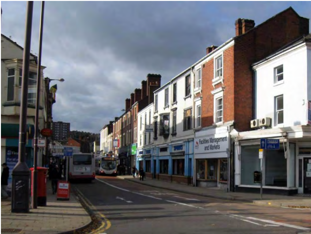
Image 25: Continuous building line to back of pavement on Church Street encloses the street – note the first floor bay windows and original shop front to corner with Glebe Street
