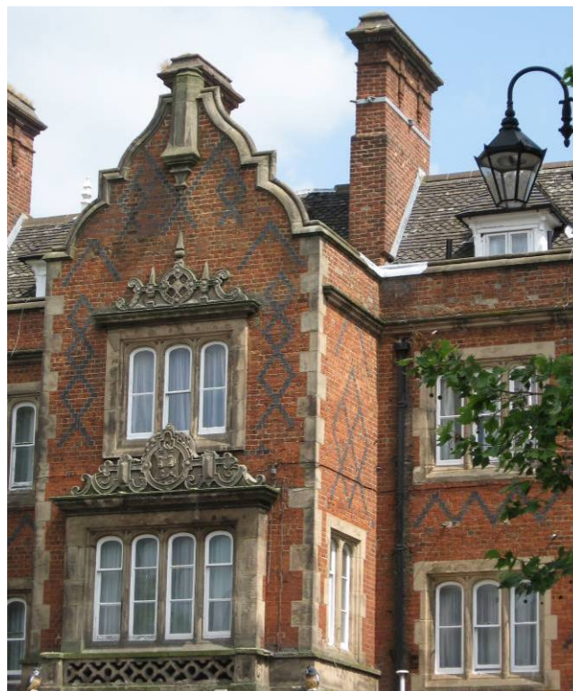
FIGURE 11: Decorated stone detailing to the central advanced bay of the hotel
