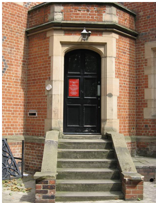
FIGURE 14: Corner porch and front door to one of the former residential buildings
