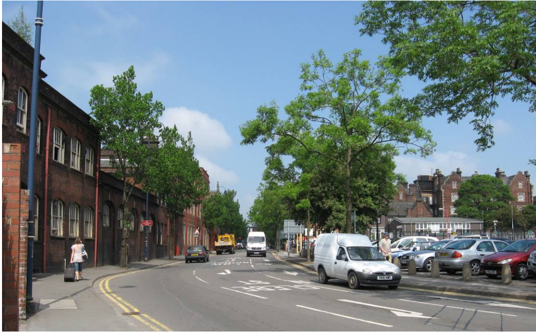
FIGURE 5: View towards the Conservation Area with the station complex on the left
