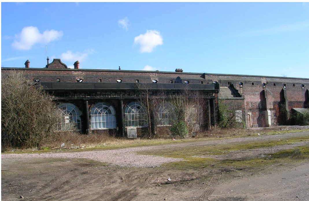
FIGURE 19: The rear of the station
