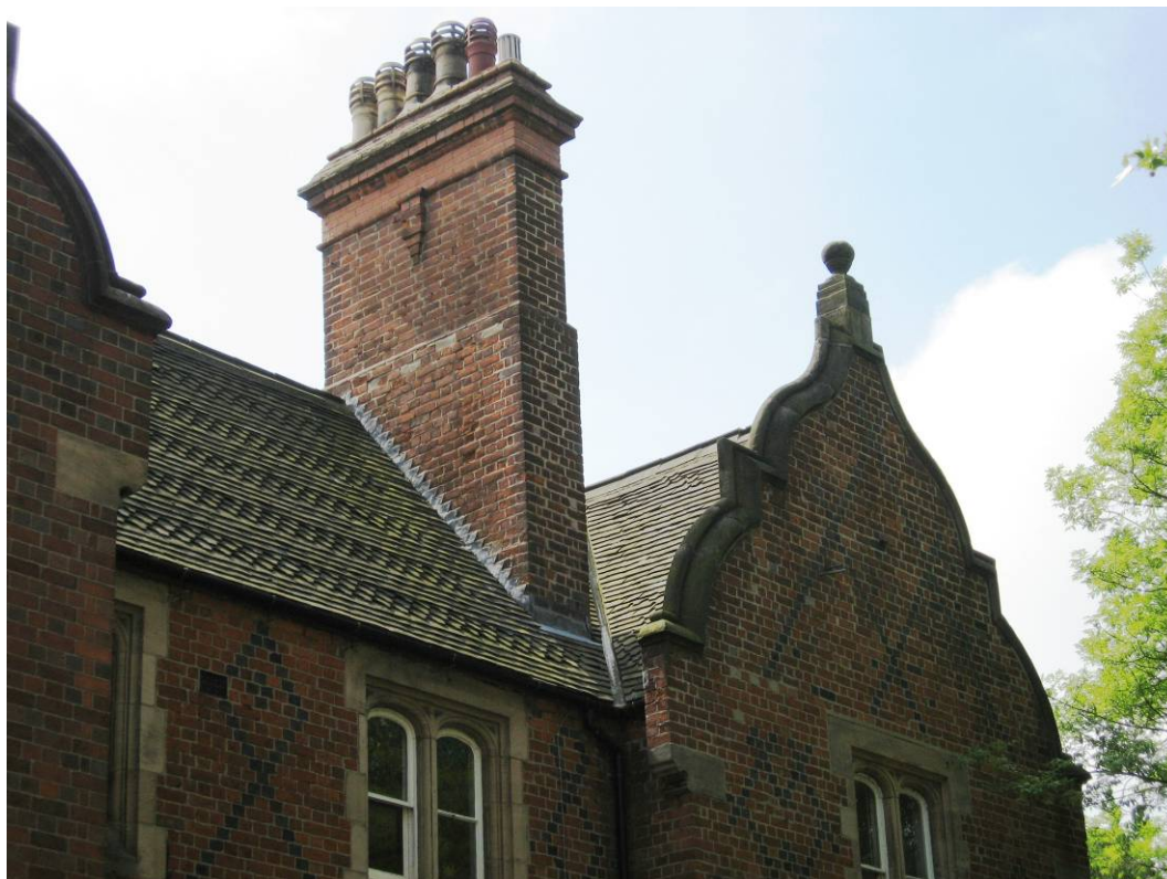
FIGURE 12: Roof and chimney stacks on one of the former residential buildings
