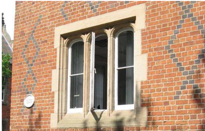
FIGURE 13: Stone mullioned casement window to one of the former residential buildings
