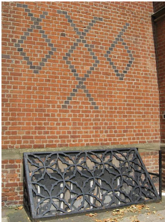
FIGURE 9: Diaperwork and metalwork detailing common throughout the square
