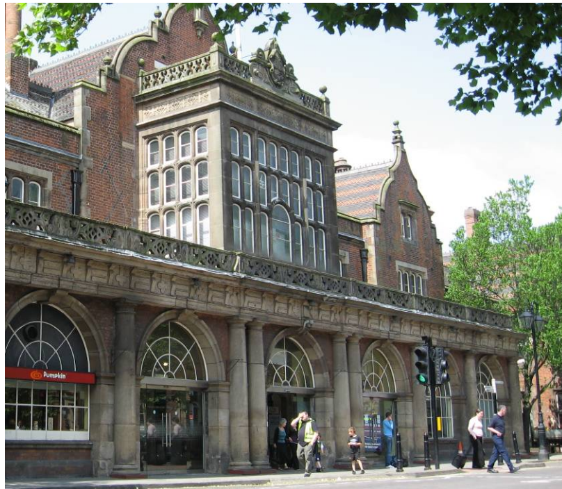
FIGURE 10: The front entrance to the station
